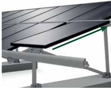
Shift the module upwards into the rail
